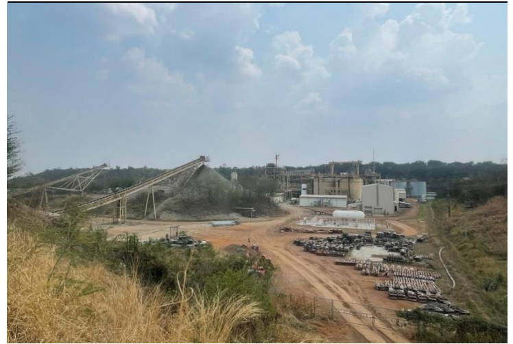
Figure 32: Chatree processing plant (>5Mtpa capacity over two plants) – currently processing low grade stockpiles
